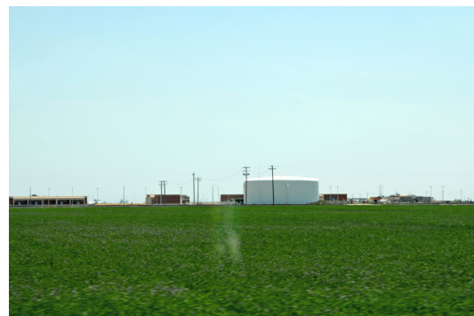
A water storage tank near West Hills College.
