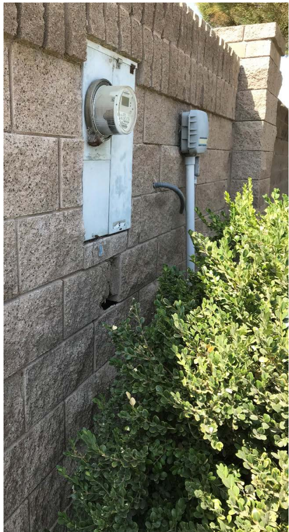
Block wall on Silverado Drive
