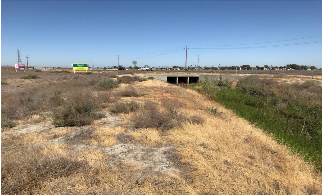
Photograph 3: View along Ditch 10 to box culvert under State Route 198. 36.2578, -119.8627, view west. Photograph taken by Dylan Ayers on June 14, 2018.
