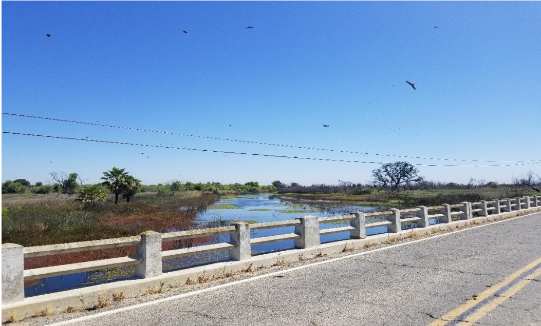
Photograph 13: Kings River, bridge, and cliff swallows east of Project. 36.2557, -119.8552, view southwest. Photograph taken by Dylan Ayers on June 14, 2018.
