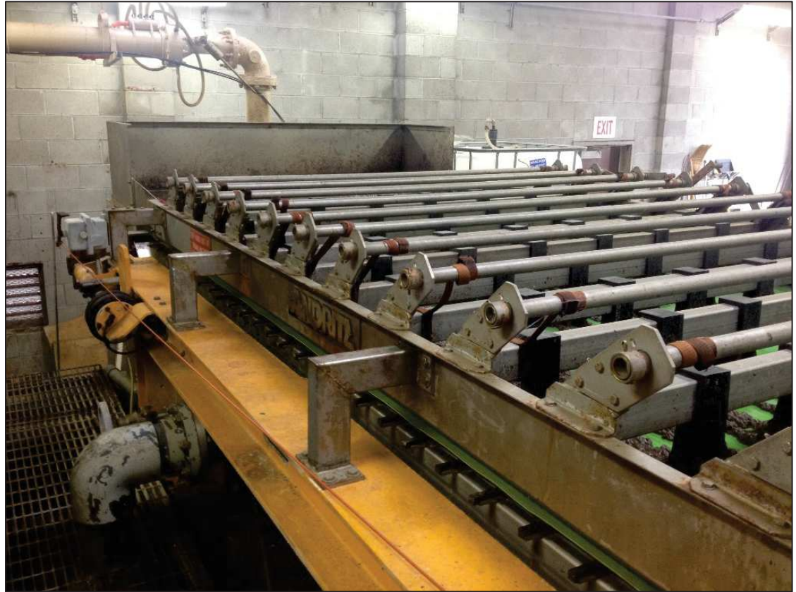
Figure 9.8 Example of Gravity Belt Thickening
