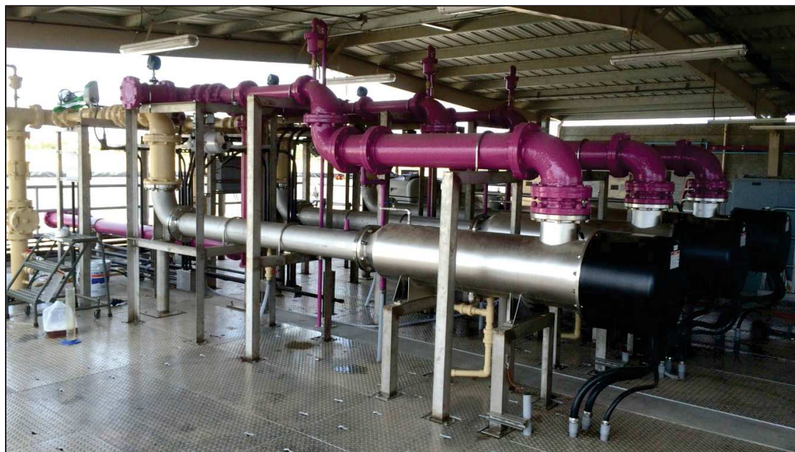
Figure 9.6 Example of In-Vessel UV Disinfection
