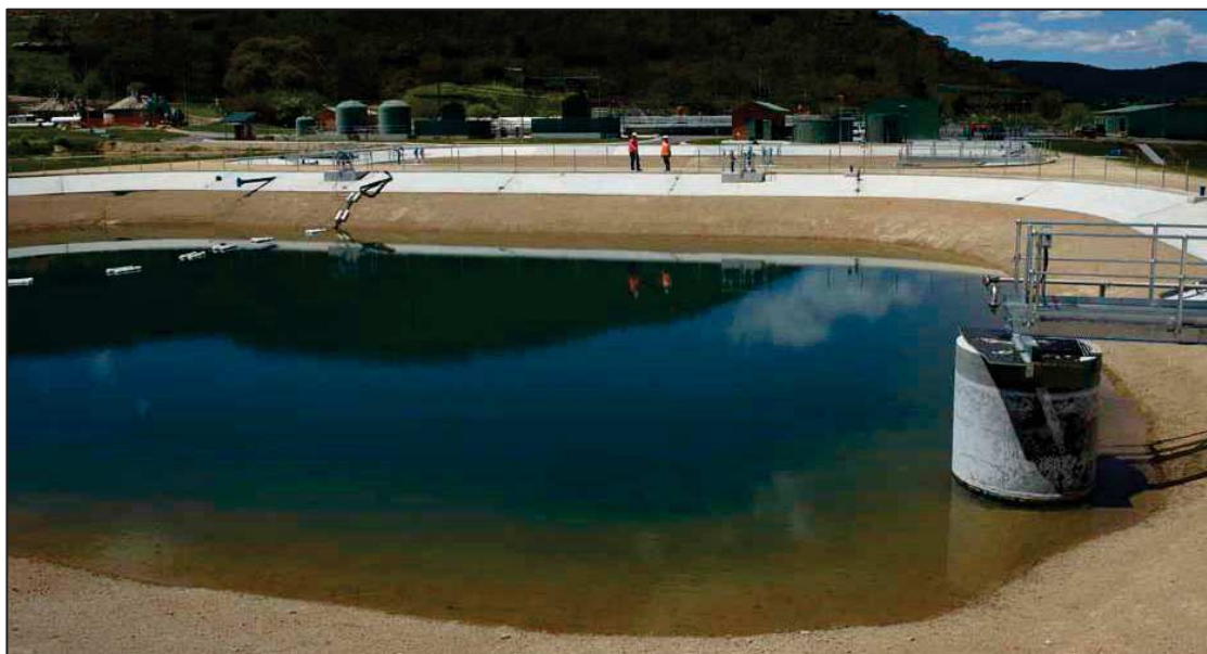
Figure 9.10 Example of Solids Lagoon Stabilization
