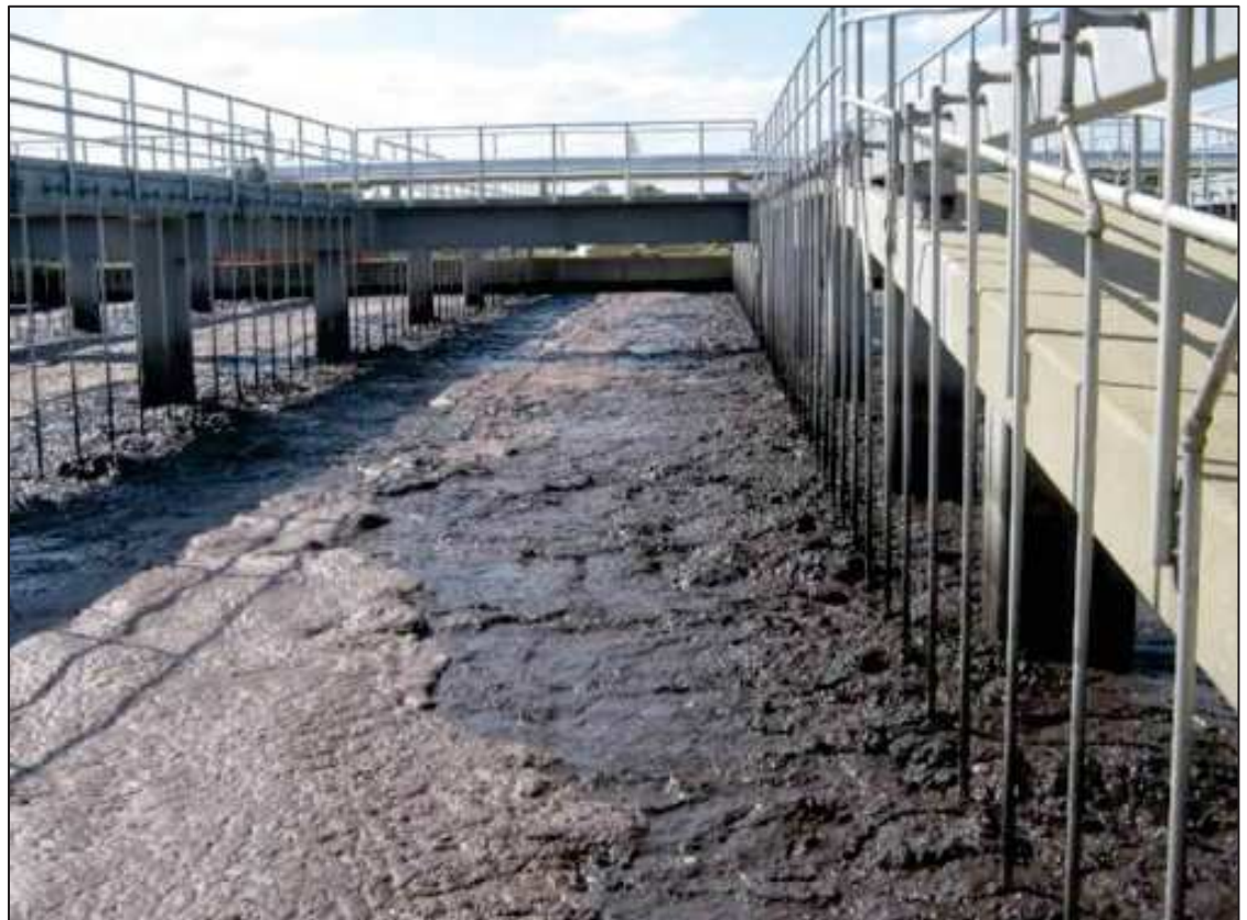
Figure 9.9 Example of Aerobic Digestion Solids Stabilization
