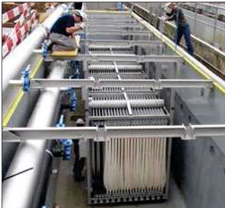
Figure 9.5 Example of a Membrane Bioreactor Secondary Treatment Process.
