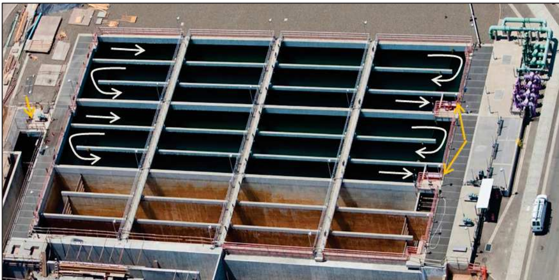
Figure 9.7 Example of Chlorine Contact Basin Disinfection
