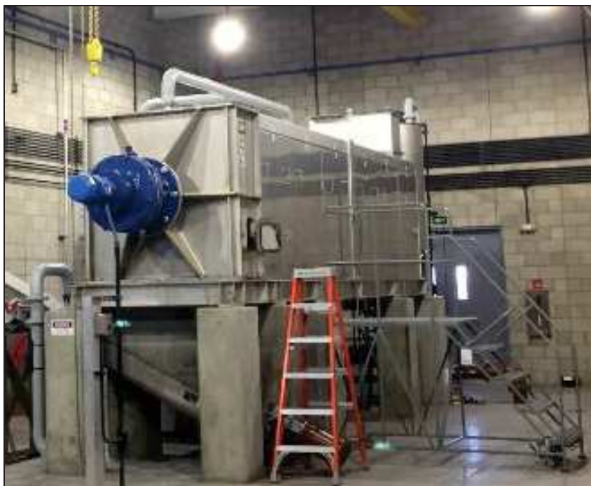
Figure 9.11 Example of Screw Press Solids Dewatering
