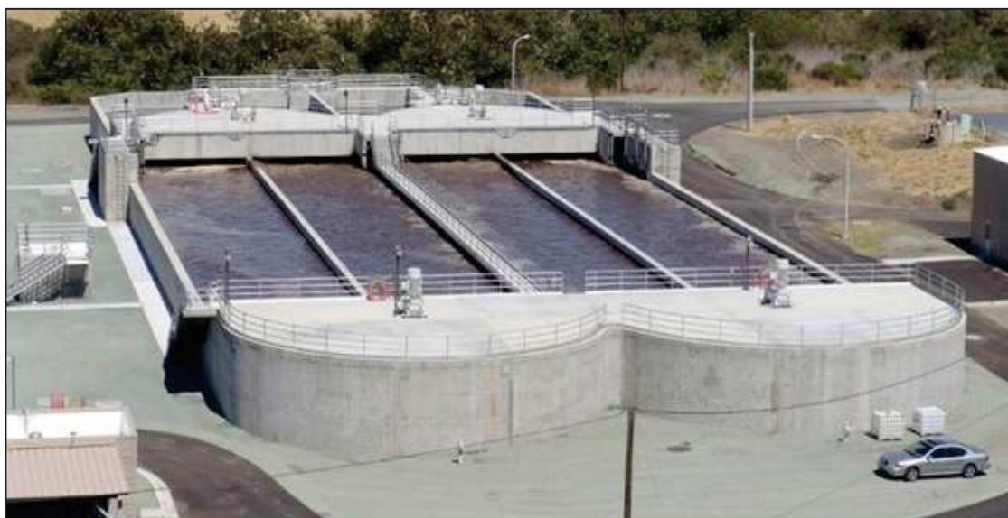
Figure 9.4 Example of an Oxidation Ditch Secondary Treatment Process.
