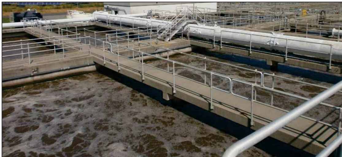
Figure 9.3 Example of a Conventional Activated Sludge with Modified Ludzack Ettinger Secondary Treatment Process.
