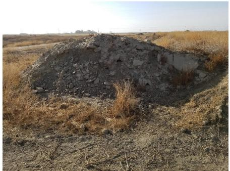
Photo 60: View of soil pile near berm of basin. The origin of these soil piles is unknown and therefore qualifies as a REC.
