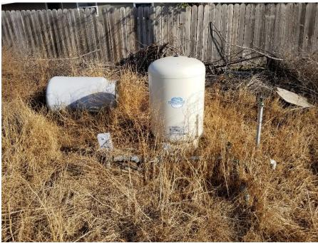
Photo 18: View of second well along western boundary of residence west of the abandoned dairy building. Although not a REC, any well that is not going to remain in use, should be abandoned in accordance with state and local regulations.
