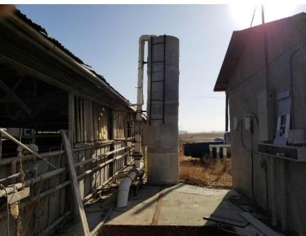
Photo 10: View of standpipe along western boundary of abandoned dairy building that empties into below grade vault. Use is believed to be either irrigational or part of stormwater collection system. The below grade vault has the potential to concentrate contaminants if used for stormwater or wastewater. This vault qualifies as a REC.
