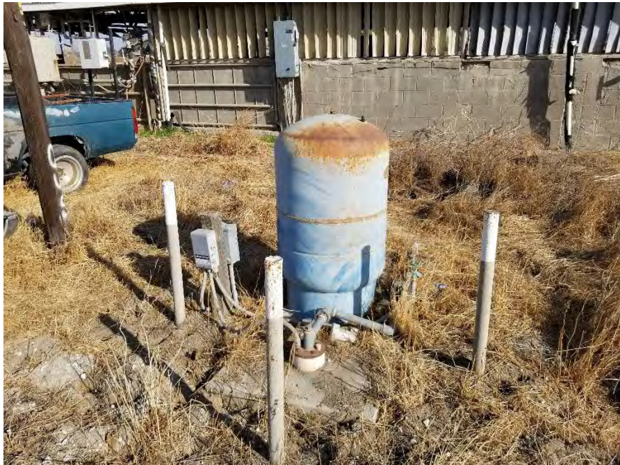
Photo 8: View of domestic well along western boundary of abandoned dairy building. The well, while not a REC, should be abandoned if not remaining in use.
