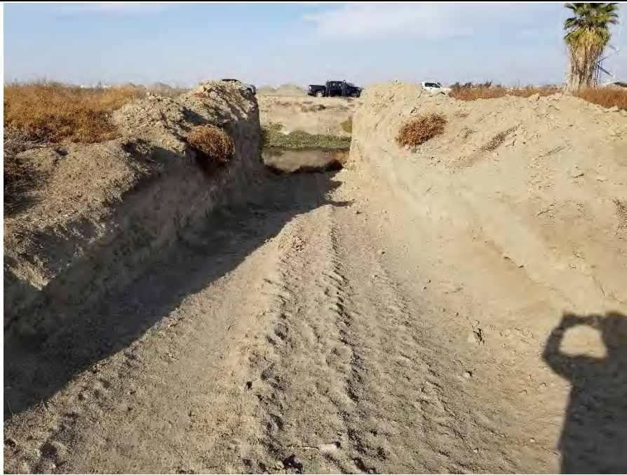
Photo 57: View of berm overflow or breach along southern boundary of the ponding basin (#4).
