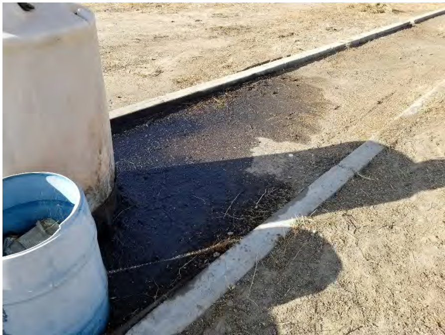
Photo 42: View of staining and spillage area from the east. Concrete and soil staining appears to be related to petroleum products. This release qualifies as a REC.
