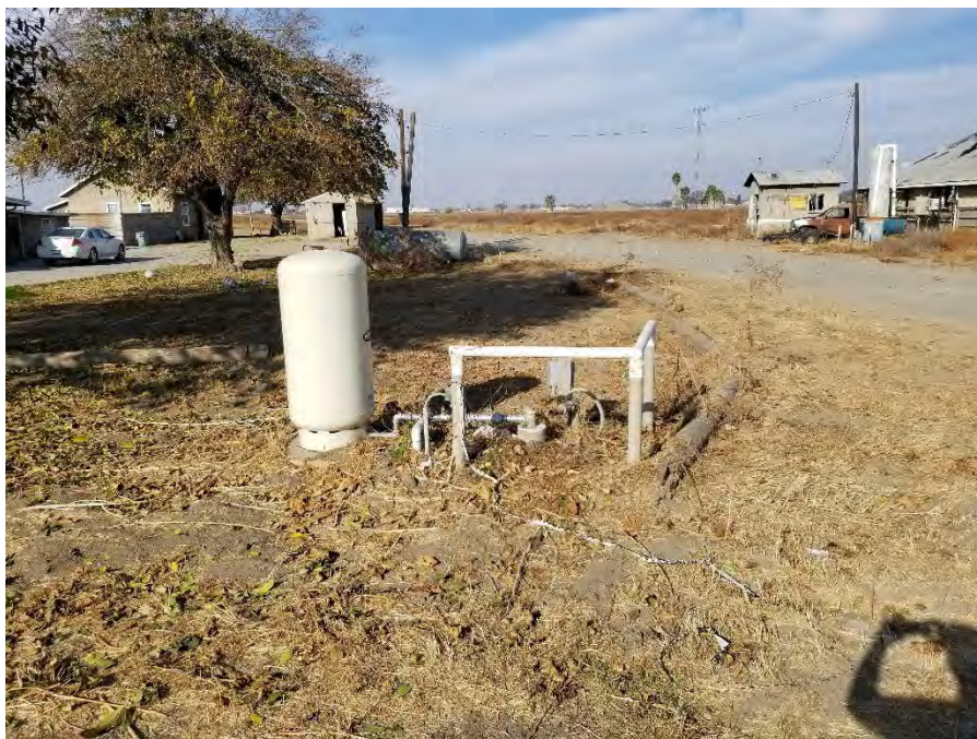
Photo 16: View of domestic well belonging to residence west of abandoned dairy building. The well is not a REC. However, any wells that are not going to remain in use should be properly abandoned in accordance with state and local regulations.
