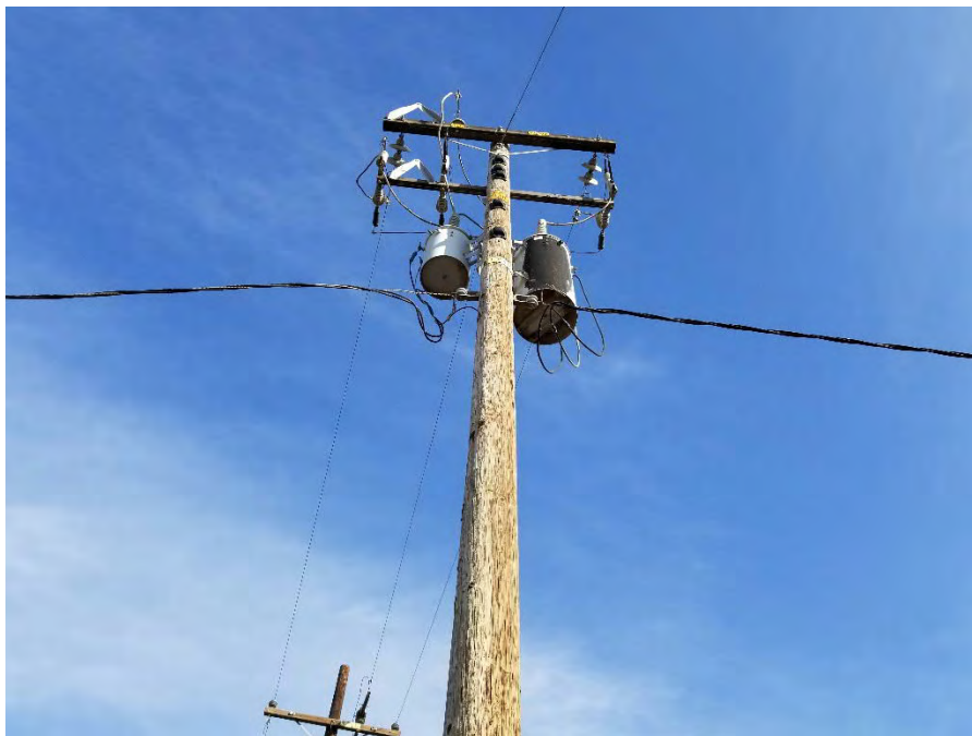
Photo 50: View of pole mounted transformers adjacent to cell tower. BSK noted staining on the right transformer. It is possible for older pole-mounted transformers to contain PCBs. These transformers qualify as a REC.
