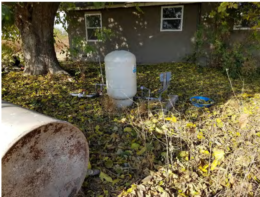
Photo 44: View of domestic well and pressure tank associated with the southernmost residence along Vine Street. Although not a REC, in the event that any well is no longer going to remain in use, it should be properly abandoned in accordance with state and local regulations. BSK did not observe any leaking or staining from the AST in the foreground. That AST should be properly disposed.
