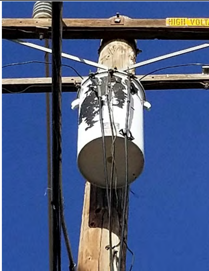
Photo 1: View of pole-mounted transformer with no signs of leaking, along western boundary of the Site. BSK could not ascertain the contents of this transformer. It is common for electrical transformers to contain PCBs. The pole-mounted transformers on the Site qualify as a REC.
